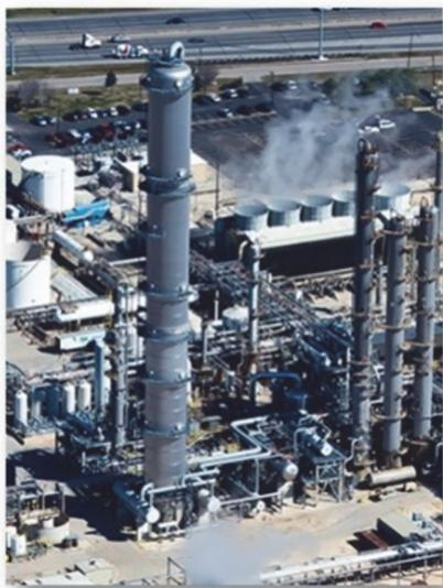
**28 ft [8.5 m] diameter x 330 ft [100 m] tall Propane/Propylene Splitter was retrofitted with SUPERFRAC® XT trays.**
