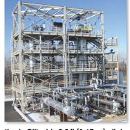
Koch-Glitsch's 5.5 ft [1.67 m] pilot plant for distillation testing with hydrocarbon mixtures.
