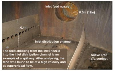
Figure 2 Existing liquid feed arrangement
