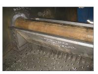
Figure 4 New liquid feed distributor
