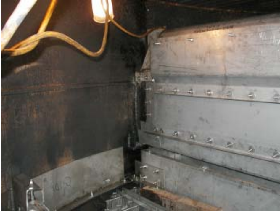
Figure 16: Flash Box Supported Using Feed Pipe and Existing Tower Attachments
