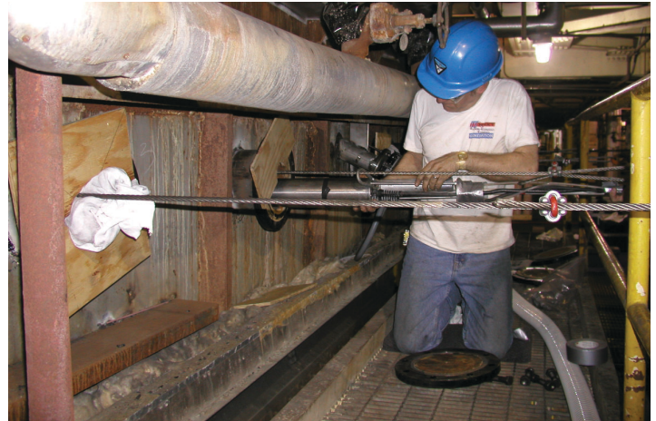
Insertion of the PDPA into a FGD scrubber.
