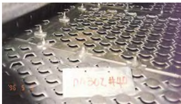
▲ Figure 14. Conventional moving-valve trays (top) in a butadiene plant had considerable fouling. The high-performance extruded fixed-valve trays (bottom) remained clean after operation.
